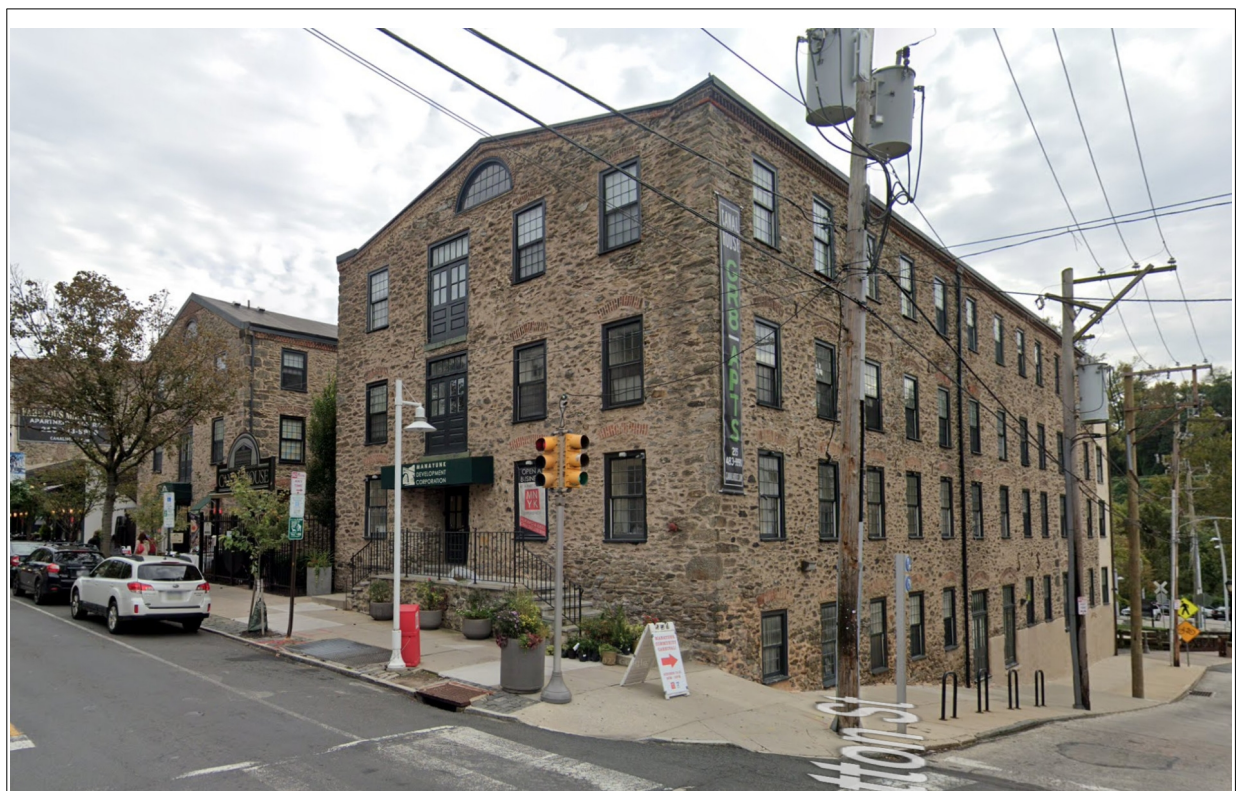
Illustration 14: Example Main Street Mills 4250 Main. Large 4-story mill building presenting as 3-story on Main Street
