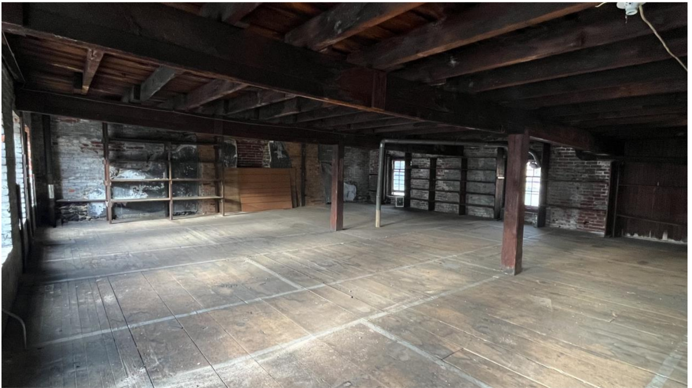
Illustration 11: Pre-1850 Historic Hotel Building 3rd Floor
