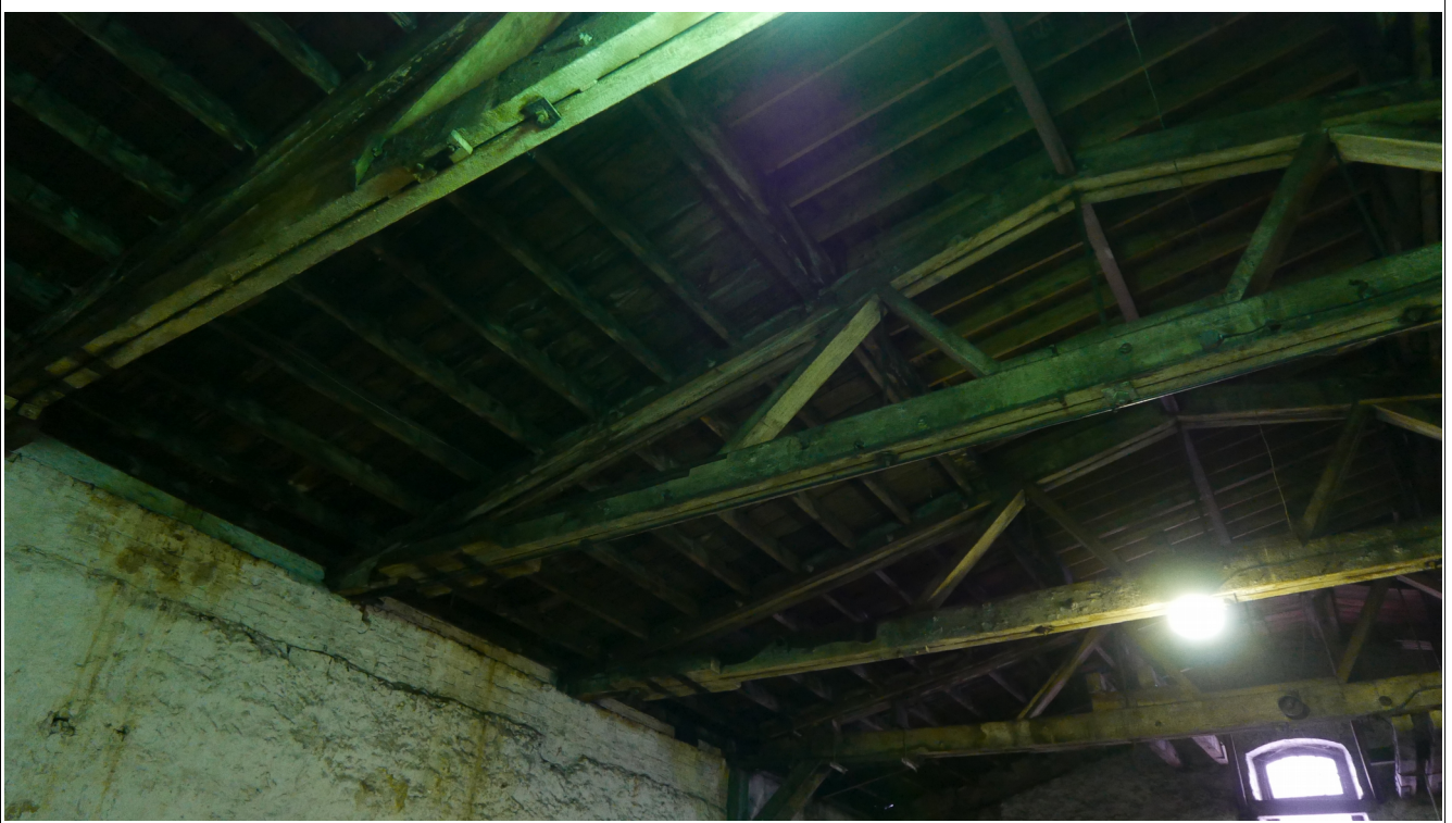
Illustration 9: Structure 8 Roof and Trusses
