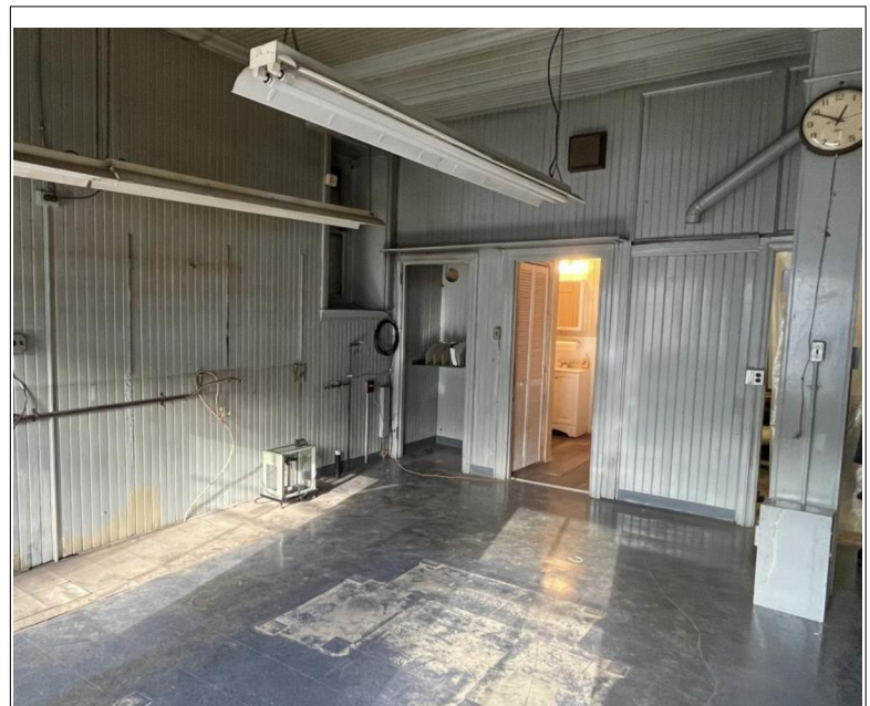
Illustration 12: Pre-1850 Historic Hotel Building 2nd Floor Office with 10' Ceilings
