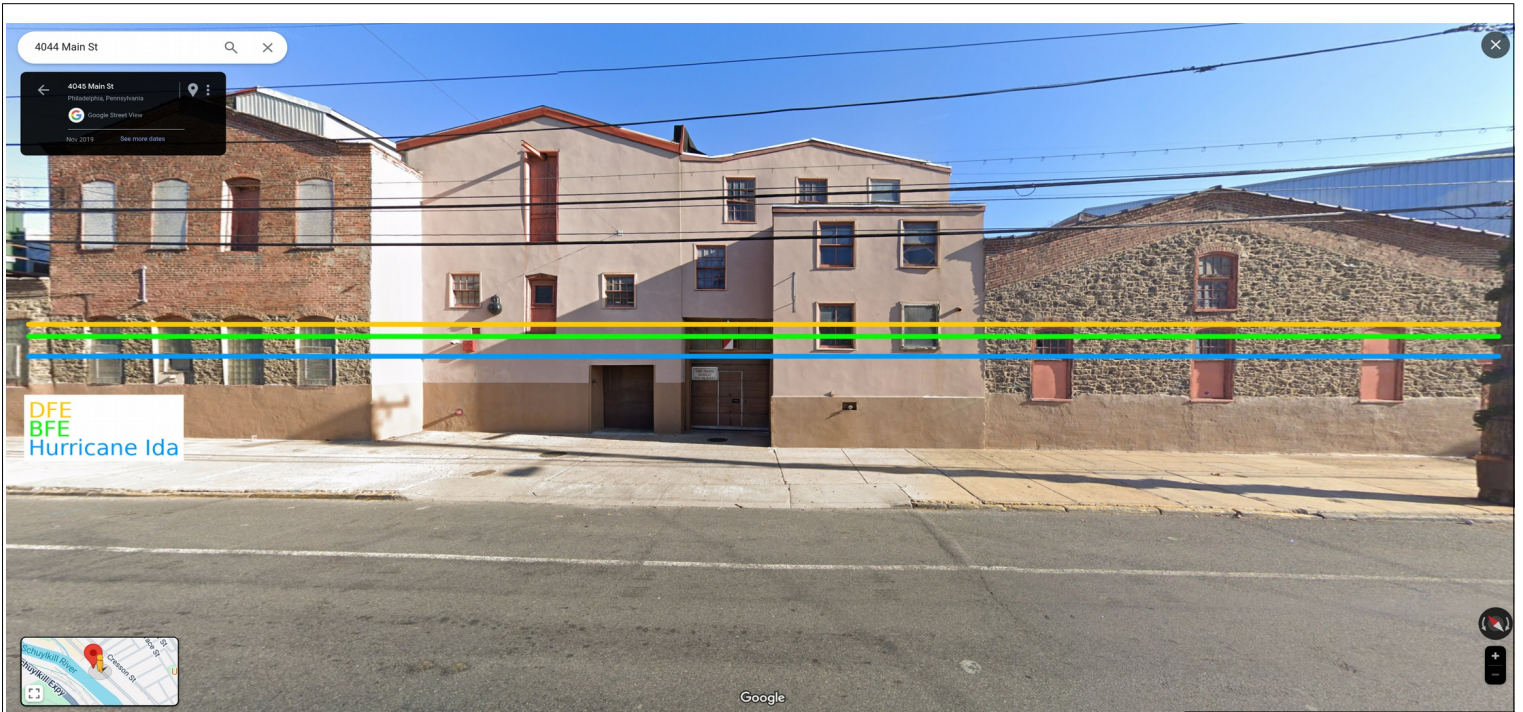
Illustration 5: Historic Mill Buildings with floors above the flood plane. Structure 8 on the right is not above the flood plain but has a beautiful historic facade and interior truss work. Ideal for a flood resistant ground level use like parking or an entrance for new construction.
