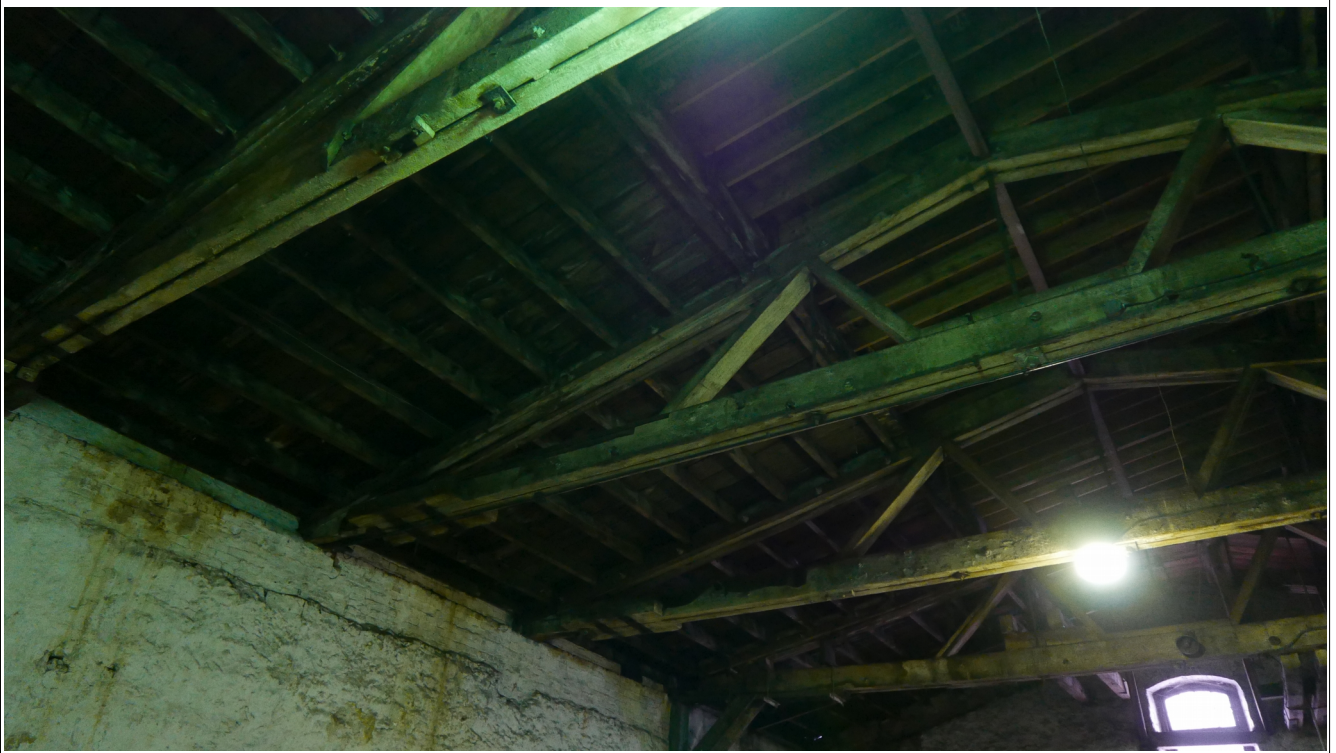
Illustration 9: Structure 8 Roof and Trusses
