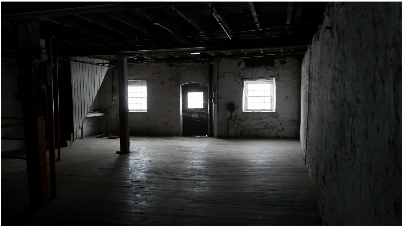
Illustration 8: Structure 7 second floor. Also a third floor above
