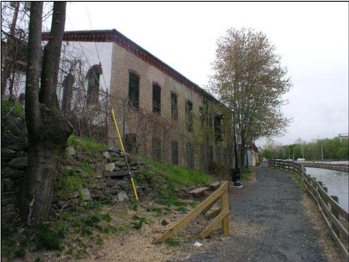
Figure 4--3 Rector Canal Access
