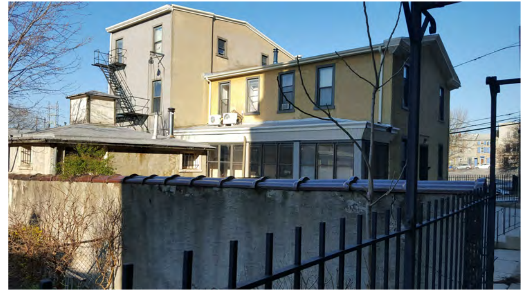
View from walkway looking north toward Convent
