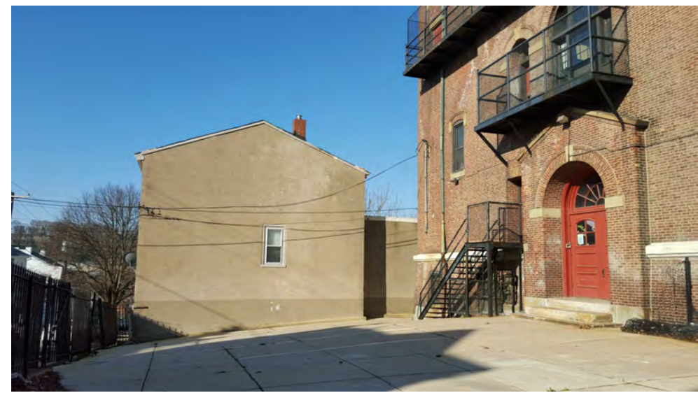
View of School and yard looking West
