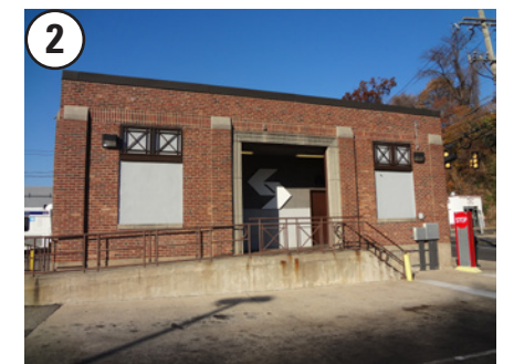
The existing Wissahickon Transportation Center building contains bathrooms and a break area, and has potential for reuse
