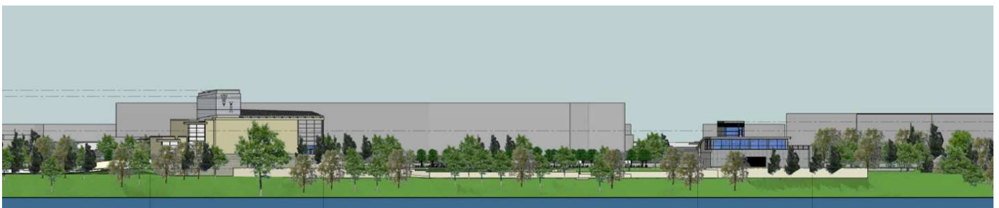
Rec Center and Tank Head House -- View from across the River
