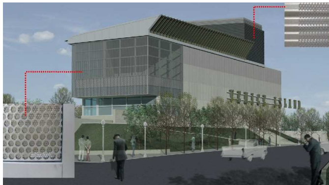
Canal side view showing construction materials
